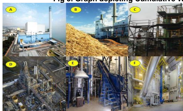
Fig 10. Some Gasification plants found around the world.
